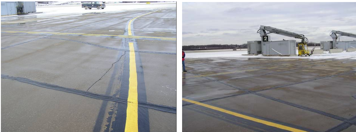
FIGURE 25. CRACKING (LEFT) AND OVERBANDED SEALANT (RIGHT) ON SAMPLE UNIT 1 OF DEICING PAD C AT AIRPORT GOLF
