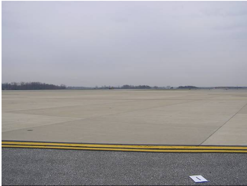
FIGURE 15. OVERVIEW OF DEICING FACILITY AT AIRPORT ECHO
