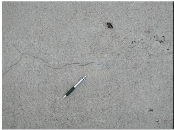
FIGURE 4. FINE HAIRLINE CRACKING OBSERVED IN SAMPLE UNIT 1 AT AIRPORT ALPHA
