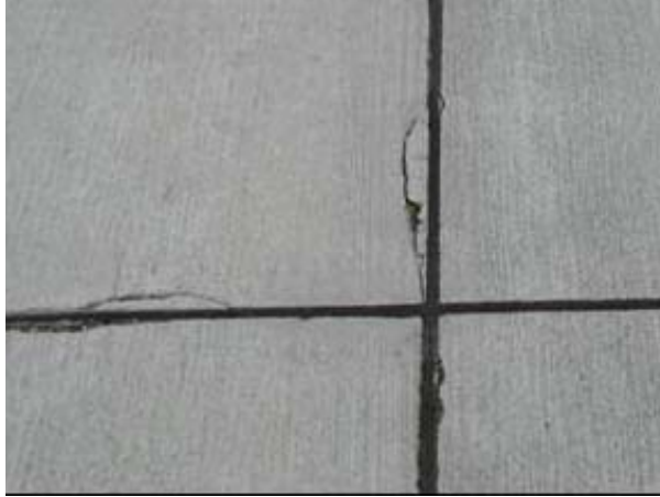
FIGURE 3. LOW-SEVERITY SPALLING (LEFT) AND LOW-SEVERITY PATCH (RIGHT) ON SAMPLE UNIT 1 AT AIRPORT ALPHA
