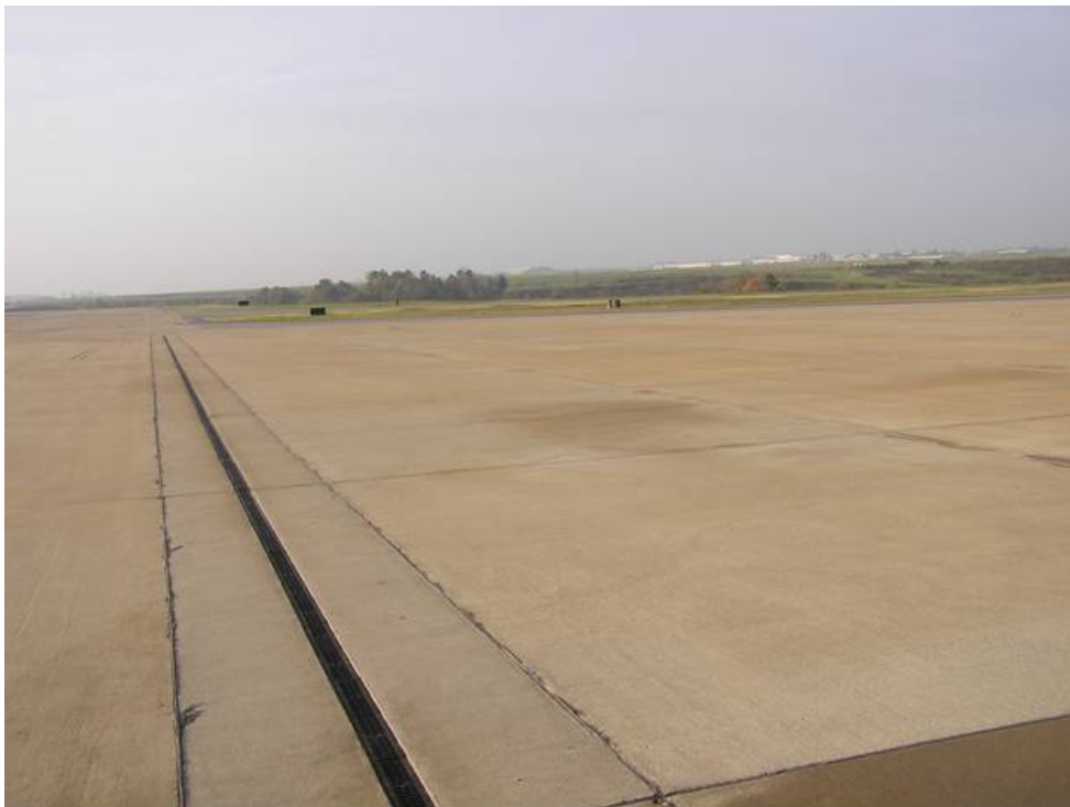
FIGURE 7. TRENCH DRAINS AROUND DEICING FACILITY AT AIRPORT BETA
