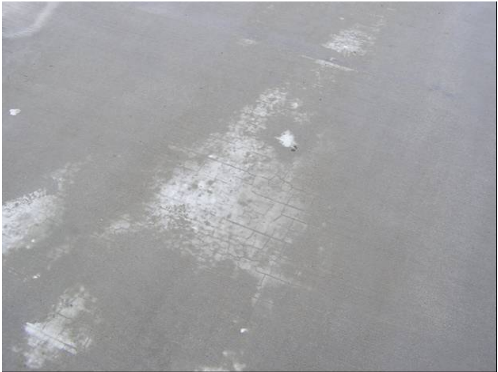
FIGURE 23. MAP CRACKING OBSERVED ON SAMPLE UNIT 1 OF DEICING PAD E AT AIRPORT GOLF
