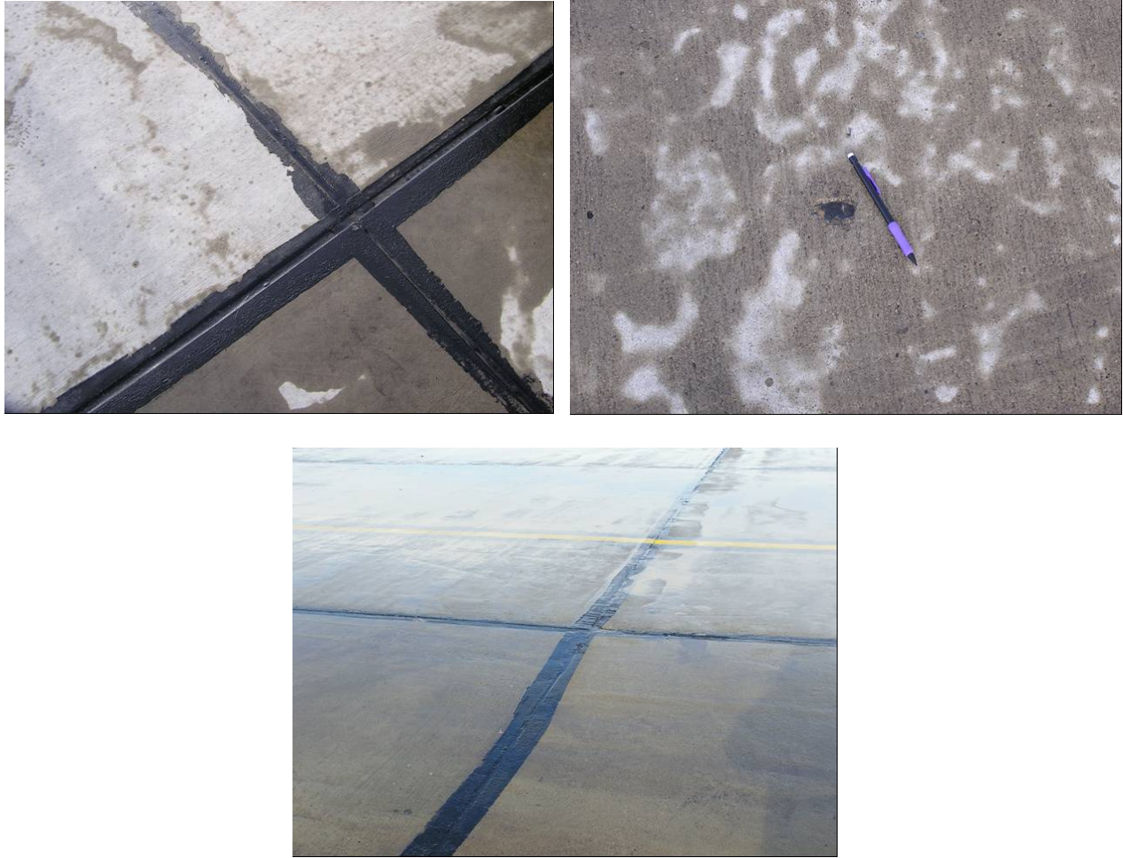
FIGURE 29. JOINT SEALANT (UPPER LEFT, SAMPLE UNIT 1), POPOUT (UPPER RIGHT, SAMPLE UNIT 2), AND OVERALL SLAB CONDITION (BOTTOM, SAMPLE UNIT 2) AT AIRPORT HOTEL
