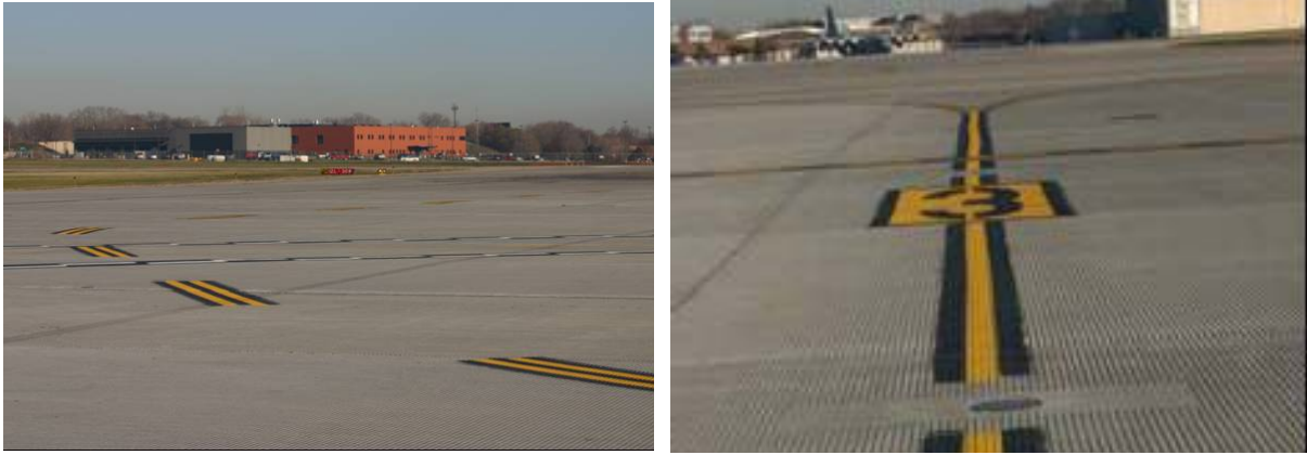
FIGURE 12. OVERVIEW OF DEICING FACILITY AT AIRPORT DELTA
