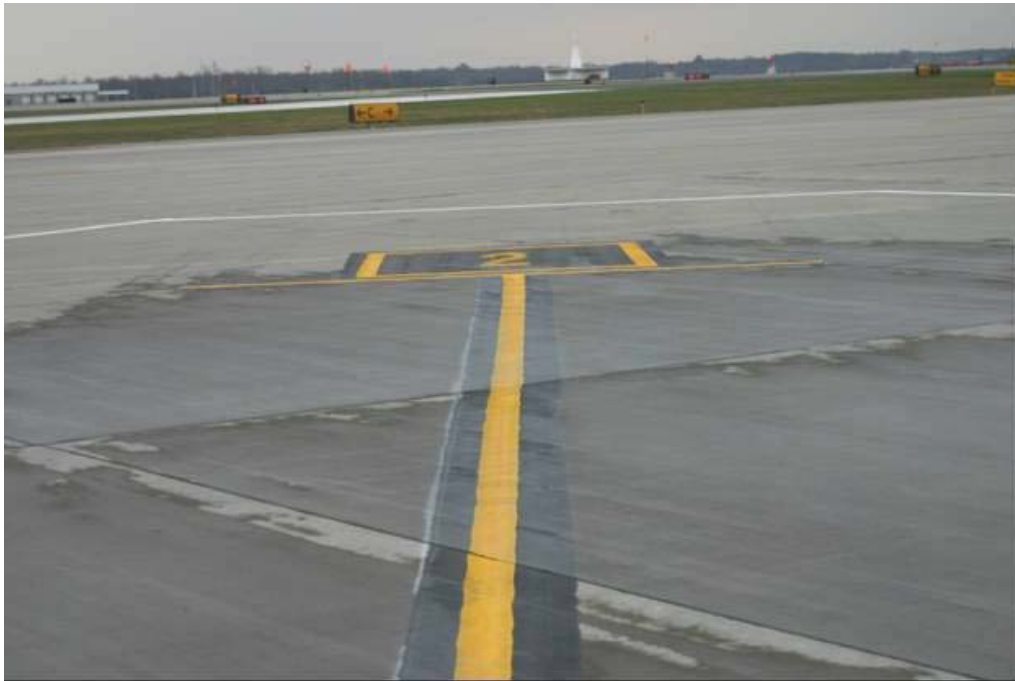
FIGURE 9. OVERVIEW OF DEICING FACILITY AT AIRPORT CHARLIE
