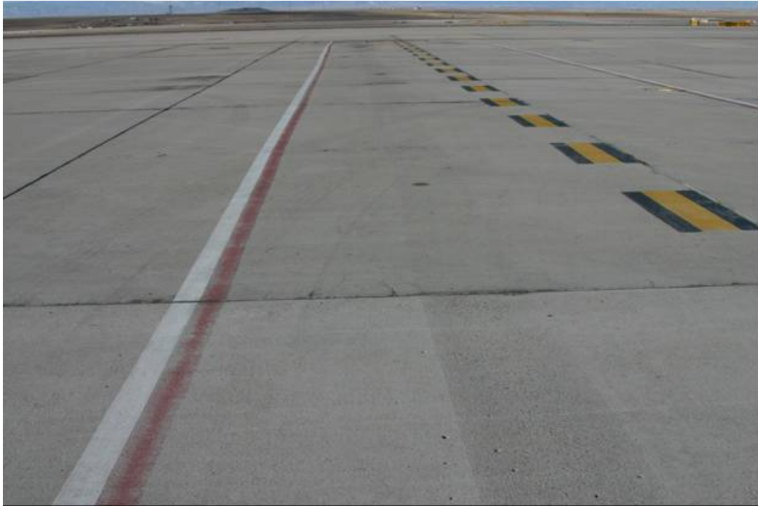
FIGURE 17. OVERVIEW OF DEICING FACILITY AT AIRPORT FOXTROT
