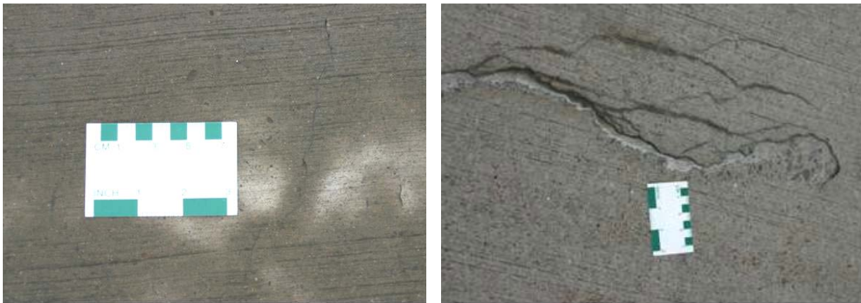
FIGURE 10. HAIRLINE CRACKING OBSERVED IN SAMPLE UNIT 1 AT AIRPORT CHARLIE
