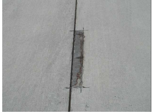
FIGURE 3. LOW-SEVERITY SPALLING (LEFT) AND LOW-SEVERITY PATCH (RIGHT) ON SAMPLE UNIT 1 AT AIRPORT ALPHA
