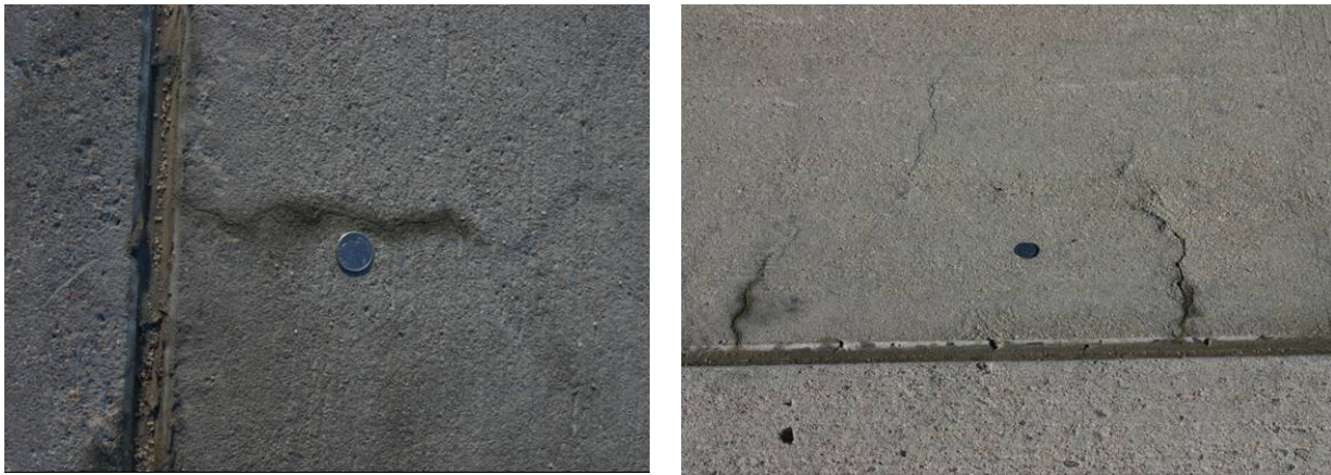
FIGURE 19. MAP AND HAIRLINE CRACKING OBSERVED ON SAMPLE UNIT 2 AT AIRPORT FOXTROT
