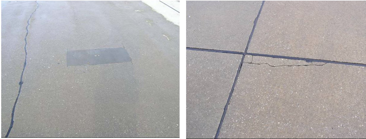
FIGURE 22. CRACKING, PATCHING, AND SPALLING OBSERVED ON SAMPLE UNIT 1 OF DEICING PAD E AT AIRPORT GOLF
