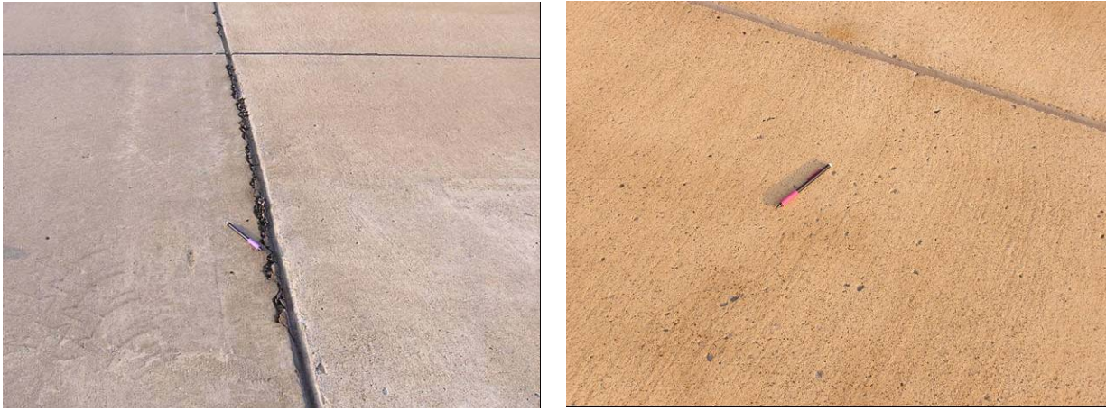
FIGURE 8. LOW-SEVERITY SPALLING (LEFT) AND HAIRLINE CRACK (RIGHT) IN SAMPLE UNIT 1 AT AIRPORT BETA
