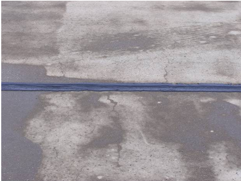
FIGURE 27. HAIRLINE CRACKING OBSERVED ON SAMPLE UNIT 2 OF DEICING PAD C AT AIRPORT GOLF
