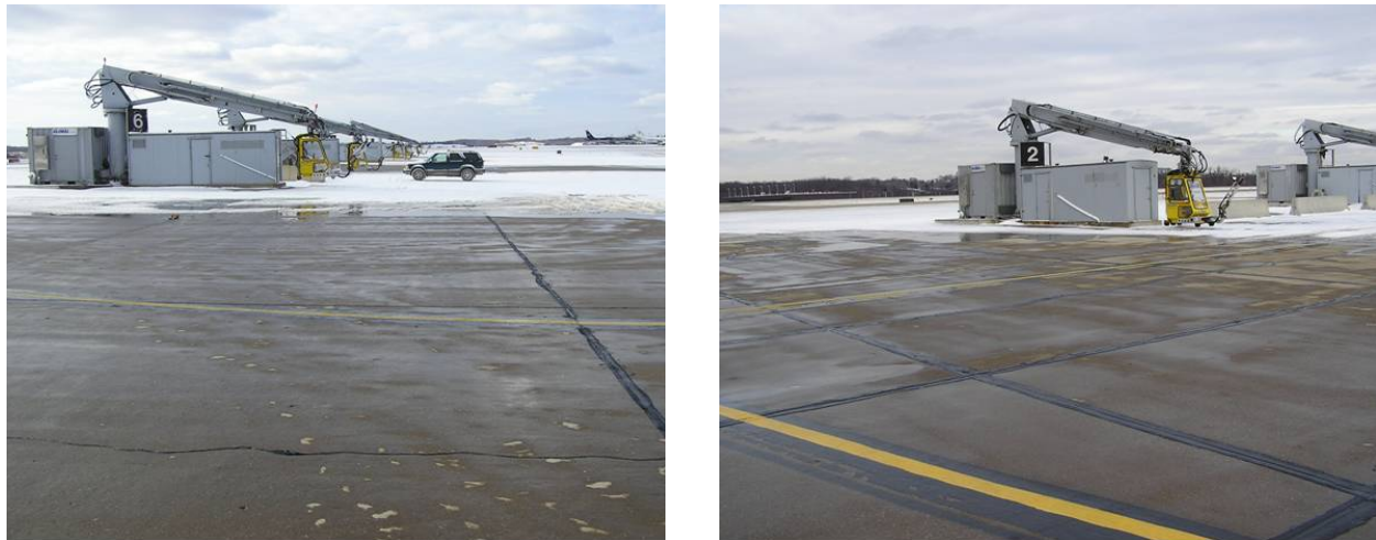
FIGURE 21. OVERVIEW OF DEICING PAD E (LEFT) AND DEICING PAD C (RIGHT) AT AIRPORT GOLF
