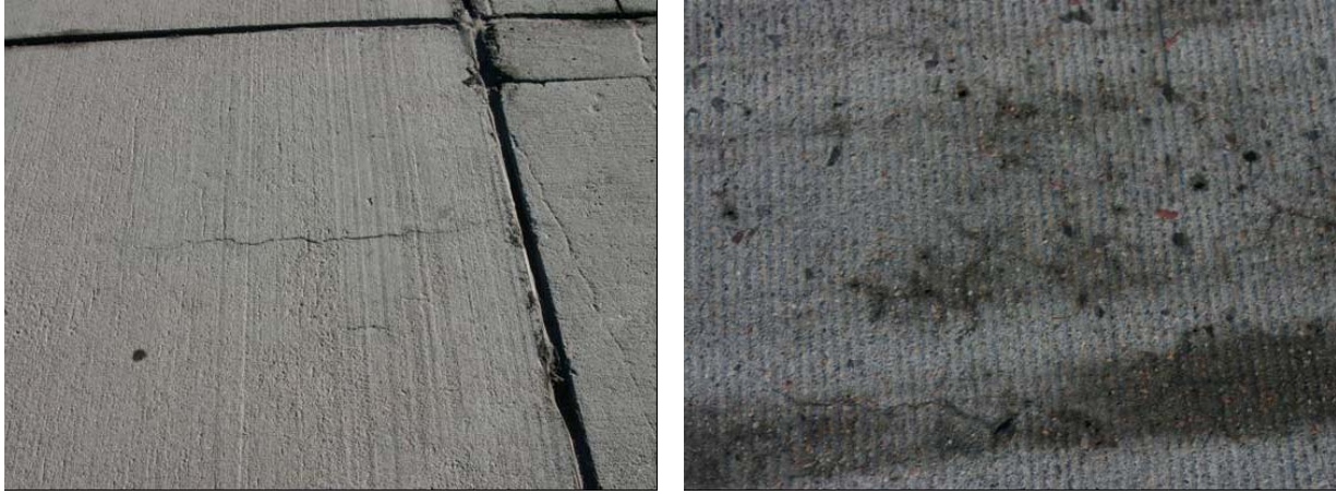
FIGURE 18. MAP AND HAIRLINE CRACKING OBSERVED ON SAMPLE UNIT 1 AT AIRPORT FOXTROT
