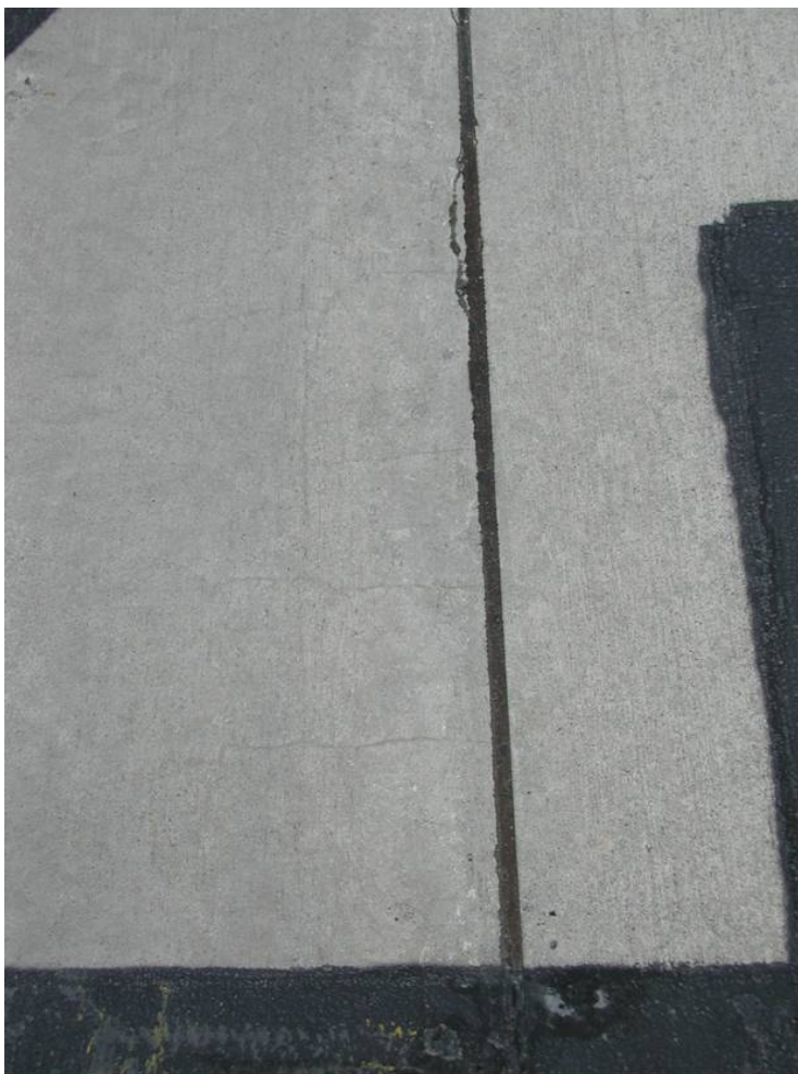
FIGURE 5. FINE HAIRLINE CRACKS NEAR A JOINT IN SAMPLE UNIT 2 AT AIRPORT ALPHA
