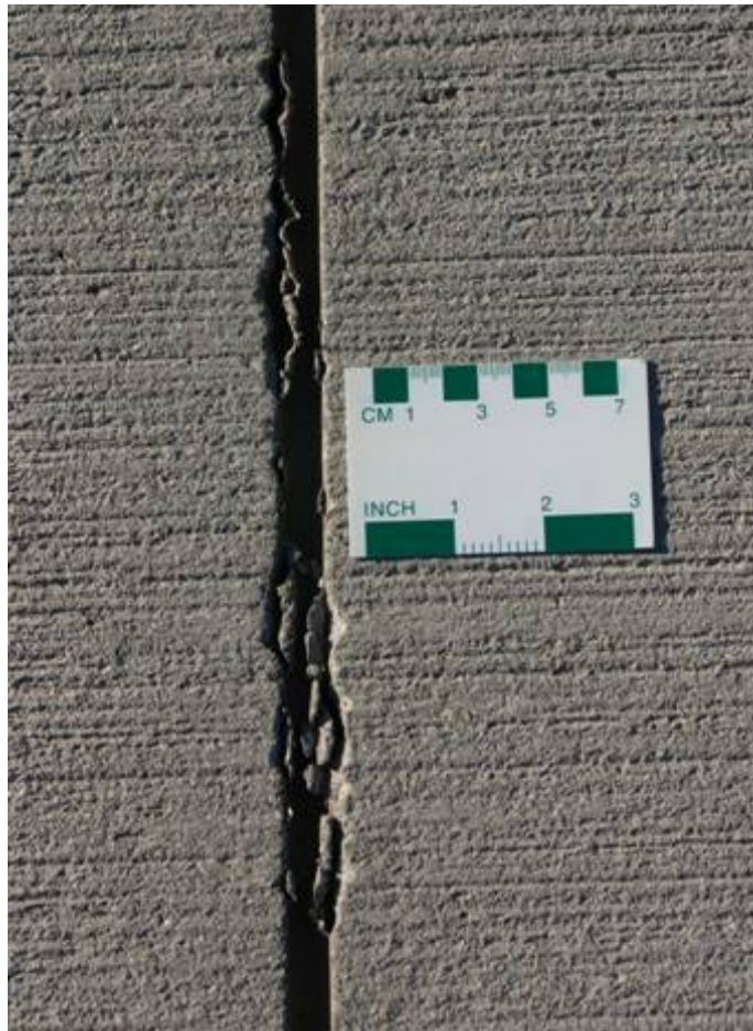
FIGURE 13. SEALANT ADHESIVE FAILURE ON SAMPLE UNIT 1 AT AIRPORT DELTA
