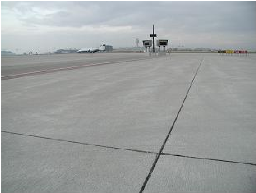
FIGURE 2. OVERVIEW OF DEICING PAD INSPECTED AT AIRPORT ALPHA
