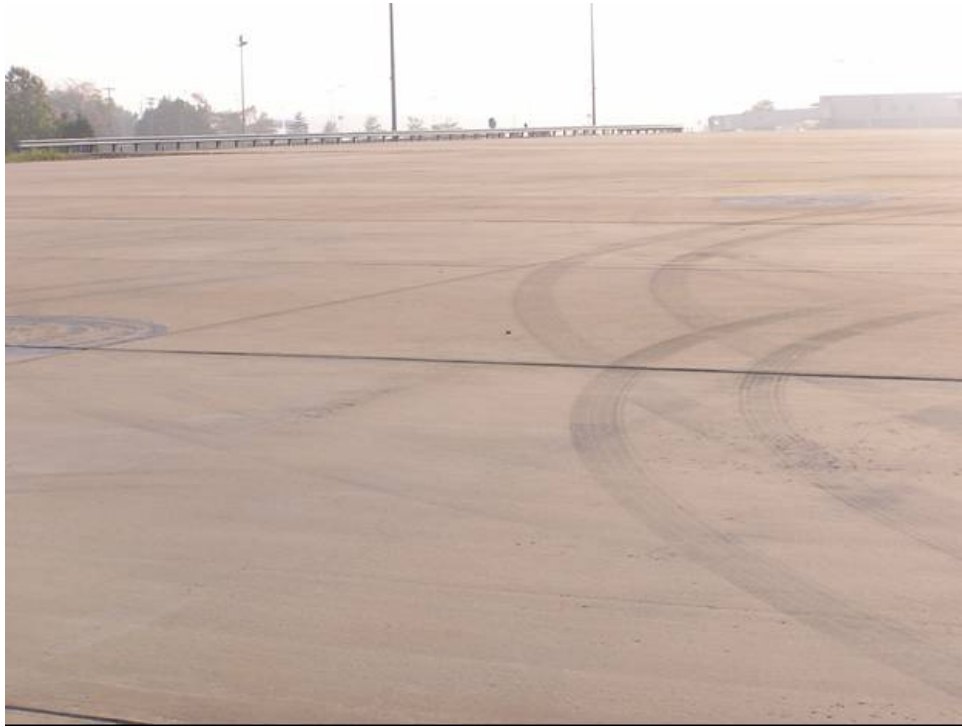
FIGURE 6. OVERVIEW OF DEICING FACILITY AT AIRPORT BETA
