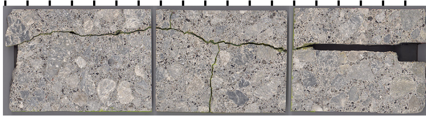
Core A, over joint, Airport Alpha
