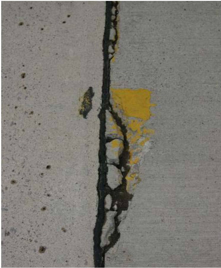
FIGURE 11. JOINT SPALLING IN SAMPLE UNIT 1 AT AIRPORT CHARLIE
