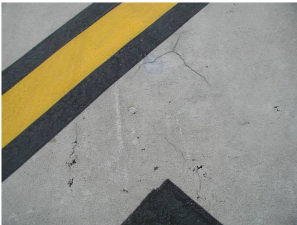
FIGURE 4. FINE HAIRLINE CRACKING OBSERVED IN SAMPLE UNIT 1 AT AIRPORT ALPHA
