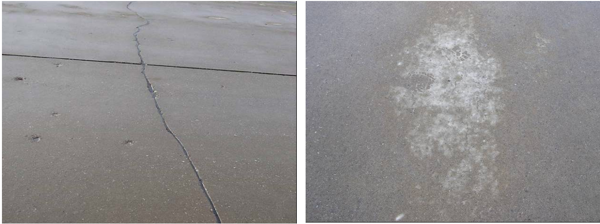
FIGURE 24. CRACKING, POPOUTS, AND MAP CRACKING OBSERVED ON SAMPLE UNIT 2 OF DEICING PAD E AT AIRPORT GOLF
