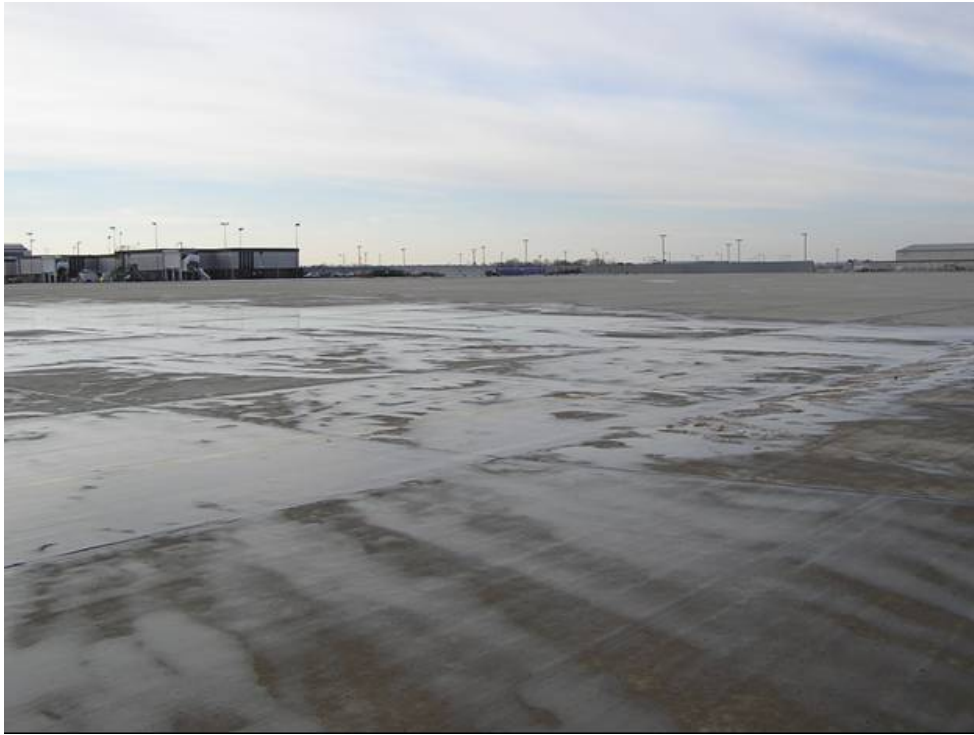
FIGURE 28. OVERVIEW OF DEICING FACILITY AT AIRPORT HOTEL
